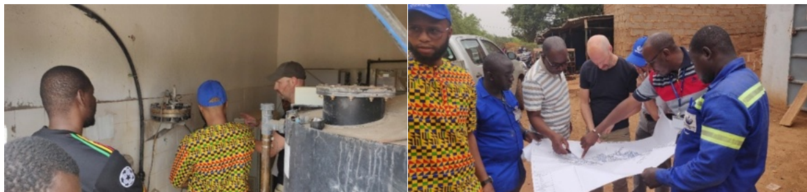
Inspecting water installation
