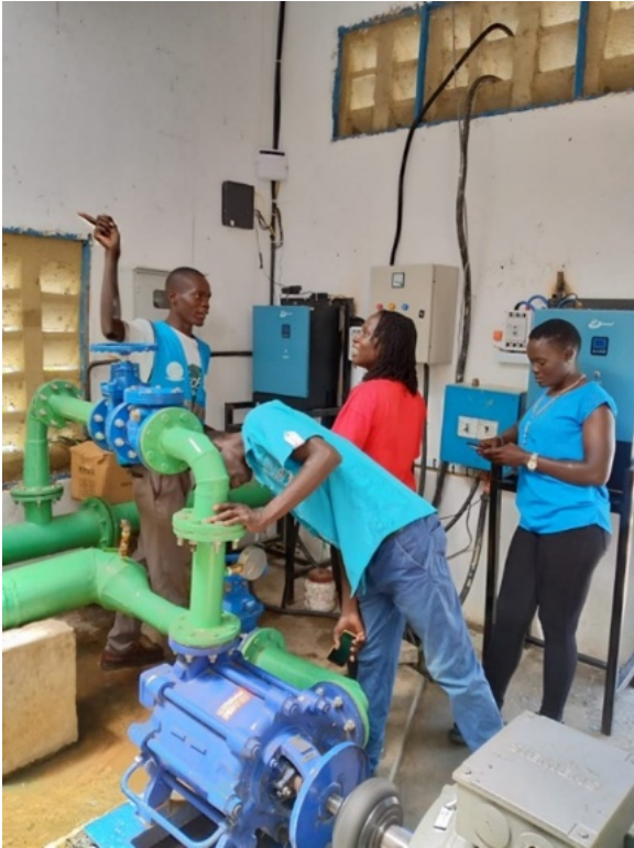
Rehabilitation of one of the water supply treatment systems
